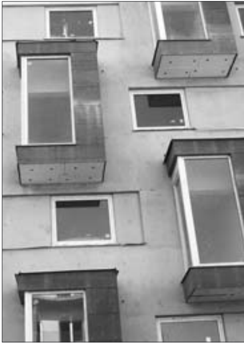
Supporting construction and anchoring of railing panels CETRIS® board 16 mm thick
