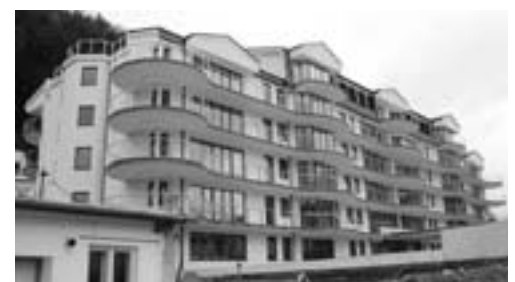
Finished structure built using the CETRIS® permanent shuttering system. ▶
